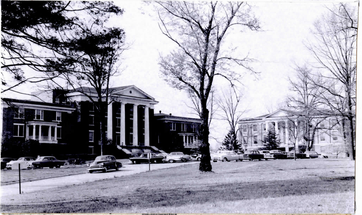
Franklin, Main, Davis, and Wright Buildings
